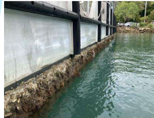
Exterior protective paint in good condition. No exterior damage to Hull.
